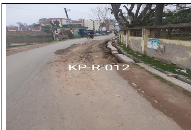
KP both road and drain Photo, KP-R-012
